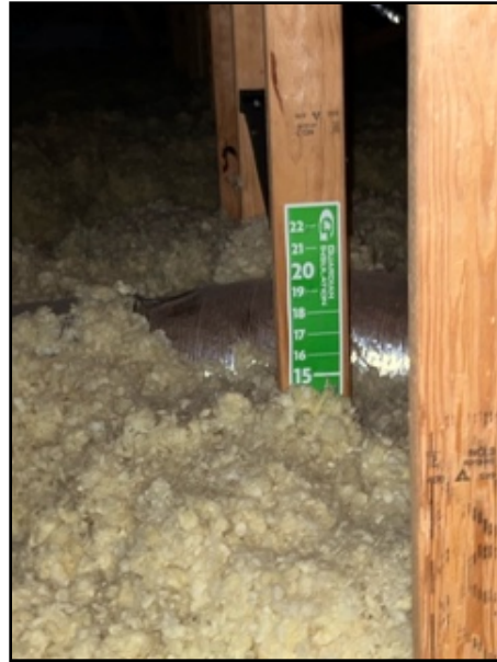
Loose Fill, Batts
